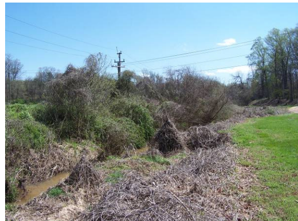
Power lines crossing Hunting Creek overhead.
