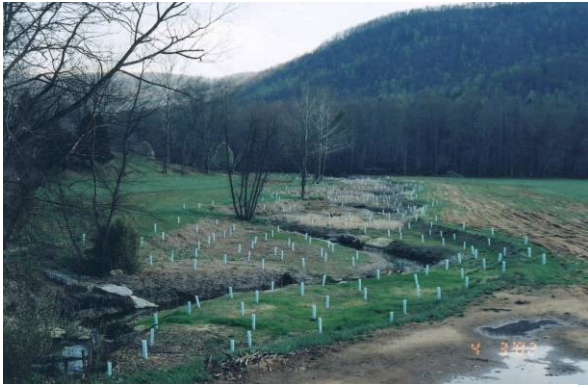
Bob's Creek with reestablished channel dimension and pattern and planted riparian area.
