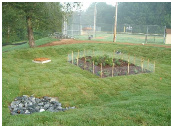
The bio-retention area is landscaped with vegetation that can withstand periodic fluctuations in water levels. It also adds to the aesthetics of the park.
