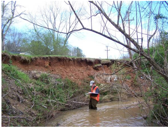
Erosion site along Hunting Creek.
