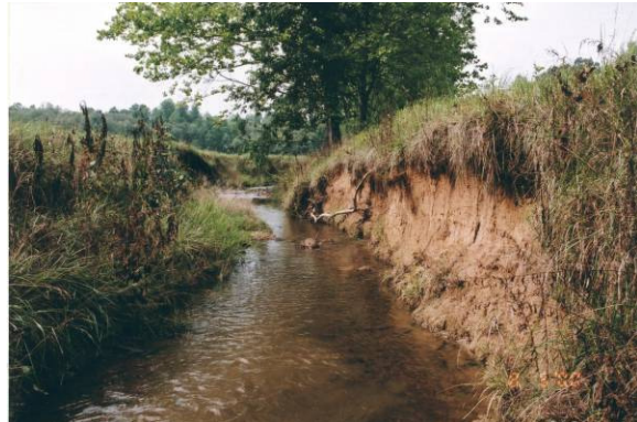
Bob's Creek, an eroding stream in the Muddy Creek Watershed that underwent stream restoration.
