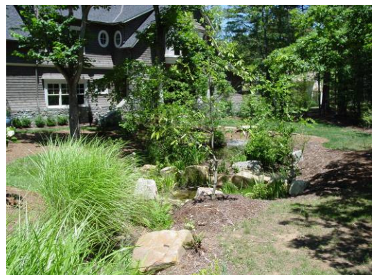
Same bio-swale as the image to the left shown 3 years after installation. In addition to treating stormwater runoff, the landscaping adds to the aesthetics of the site.
