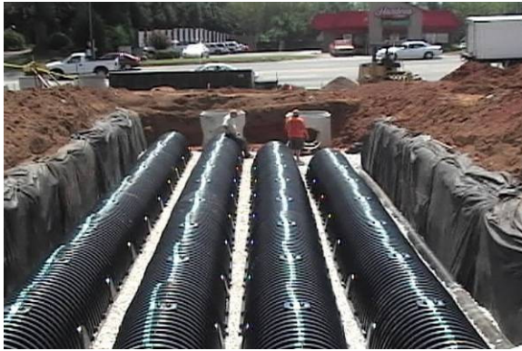
Filtration chambers are installed during construction of the Bojangles parking lot in Morganton (outside the Hunting Creek Watershed). The chambers will capture stormwater and filter it through a sand and stone medium before releasing it to a nearby stream.
