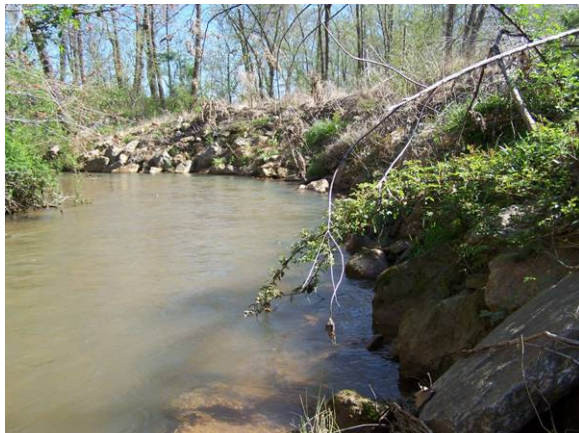
Bank armoring with rip rap along Hunting Creek.
