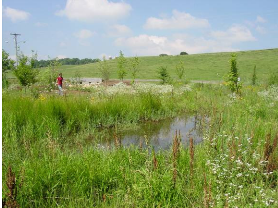
A constructed wetland at a city park captures stormwater runoff from a residential development and a parking lot. It also serves as a water feature in the park and provides wildlife habitat.
