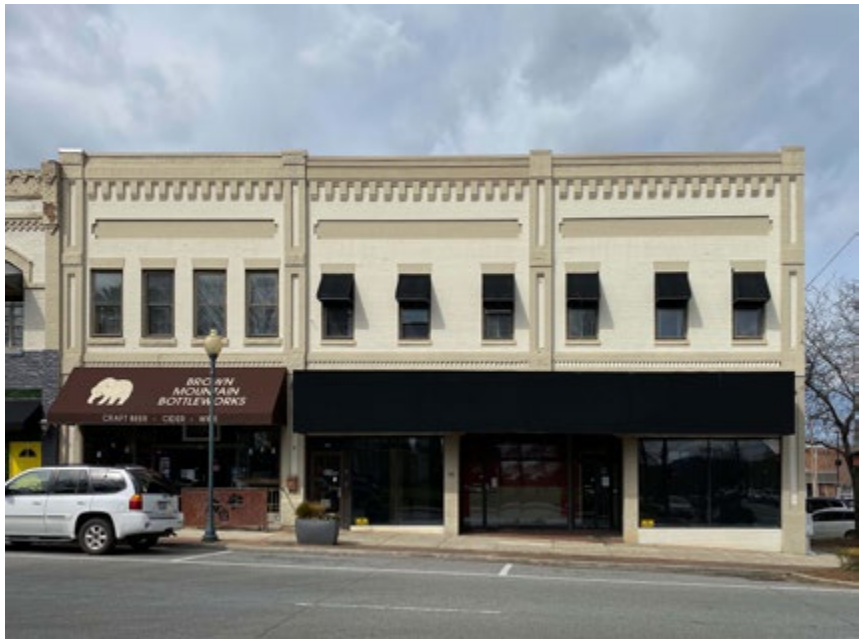
Existing Front Facade
