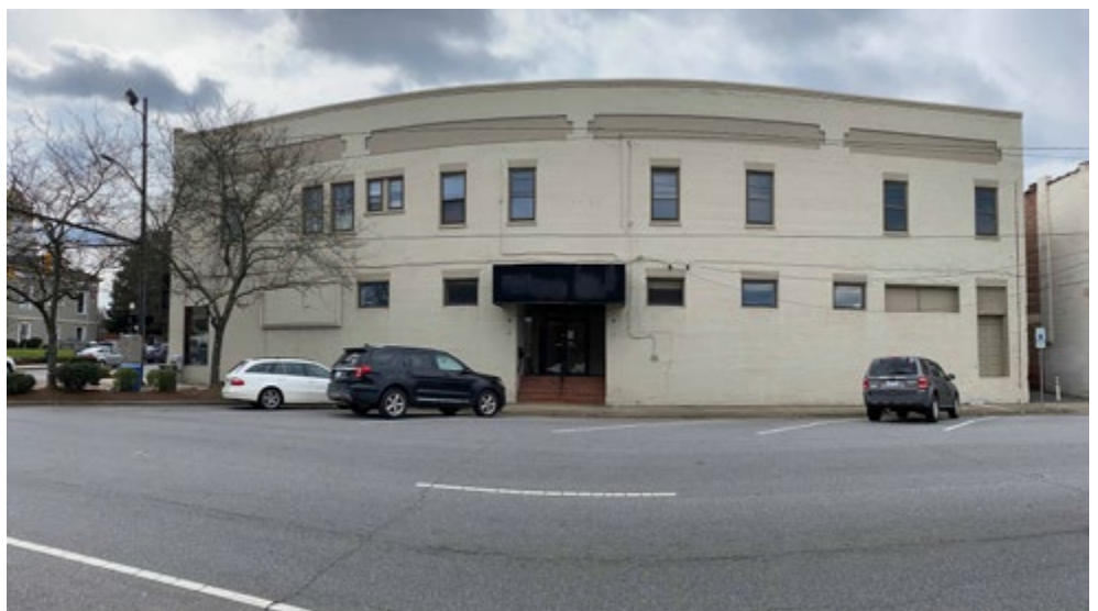
Existing Side Facade
