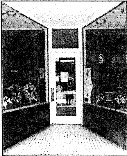
The tiled floor, large display windows, and wooden door with large glazed panel and transom of this recessed entrance are all traditional storefront features.
