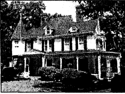
One story front porches, with turned wooden columns and rails, span the front facade and often wrap around one corner of many Queen Anne houses in Morganton. Small second story balconies are also found.
