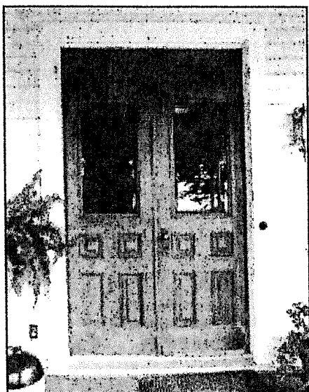
Stained, double wooden paneled front doors with glazing in the upper panels contribute to the architectural character of a Queen Anne residence.
