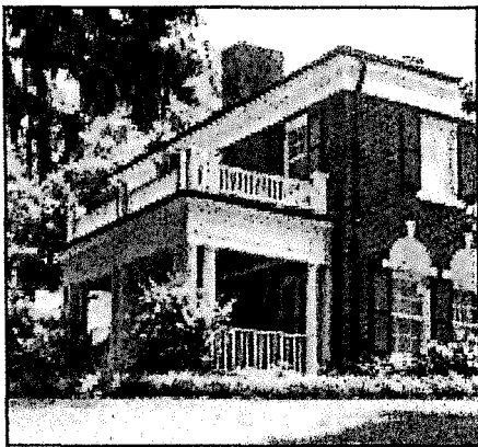
This prominent side porch, with its wide entablature and roof balustrade, is an important architectural feature of this Colonial Revival residence.
