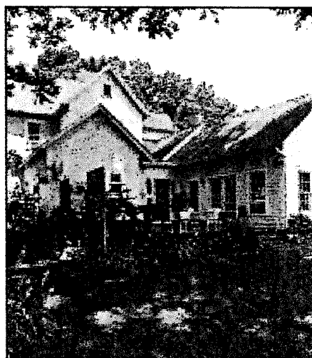
This compatible rear addition (on the right side of the photo) is subtly differentiated from the house itself by the slightly lower height of its gable roof.
