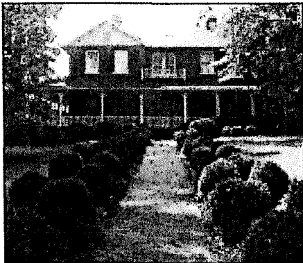
A hedge-lined brick front walk leads from the street sidewalk to the front porch of this house. Opposite page, curving concrete walkways crisscross the Broughton Hospital campus.
