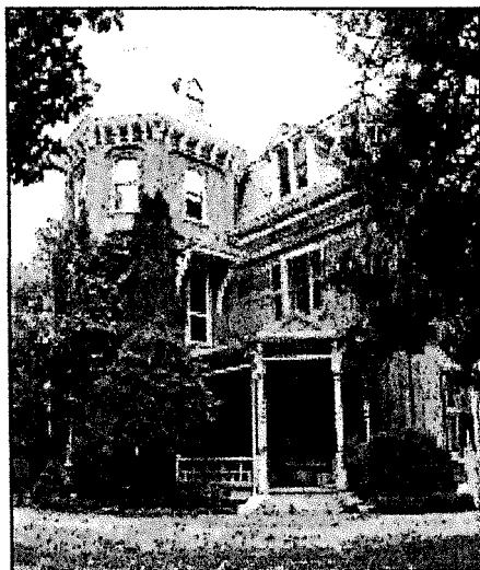
An octagonal tower and prominent wooden cornice brackets contribute to the Second Empire character of this brick residence.
