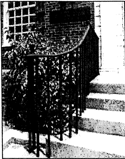
The curving form of this iron handrail illustrates one of the many shapes cast metal can take. On the opposite page, a well-detailed metal stair also meets a functional need.
