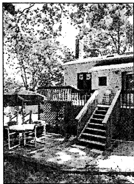
Simple, contemporary railings like these are appropriate for deck additions. Note how traditional lattice panels screen the view of the framing below this rear deck.
