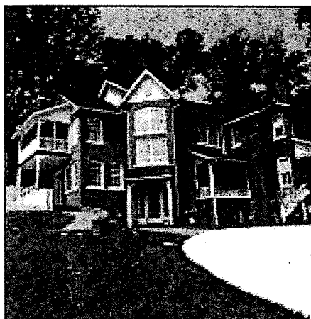
The massing of this quite substantial rear addition is minimized by the subdividing of its massing and the use of compatible materials, roof forms, and window openings.
