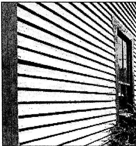
The irregular edges of deteriorated paint layers on these wood clapboards create a rough texture that should be scraped and sanded prior to repainting.
